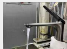
Water and leakage testing
